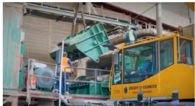
Top: Modernization of a impact hammer mill
